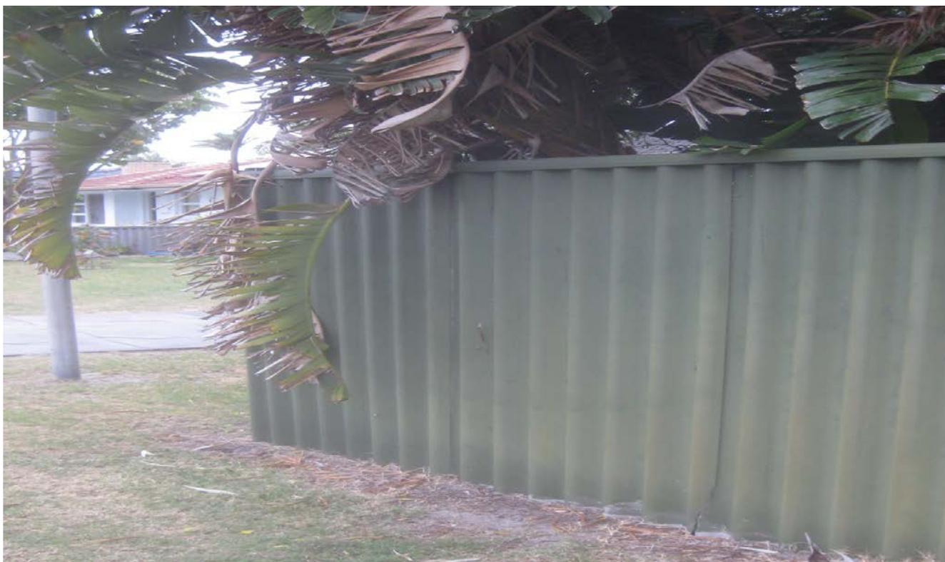
Photo 19. Painted ACM fence (with fasteners removed and with metal capping). Branches need trimming.
