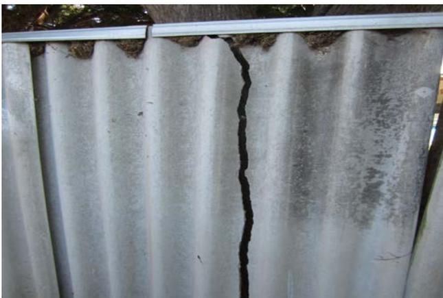
Photo 17. Cracked ACM fence
