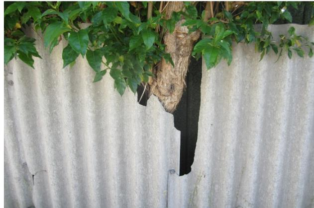
Photo 11. Tree damage to ACM fence
