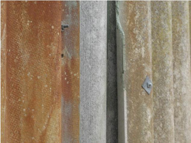
Photo 5. ACM showing hessian surface pattern
