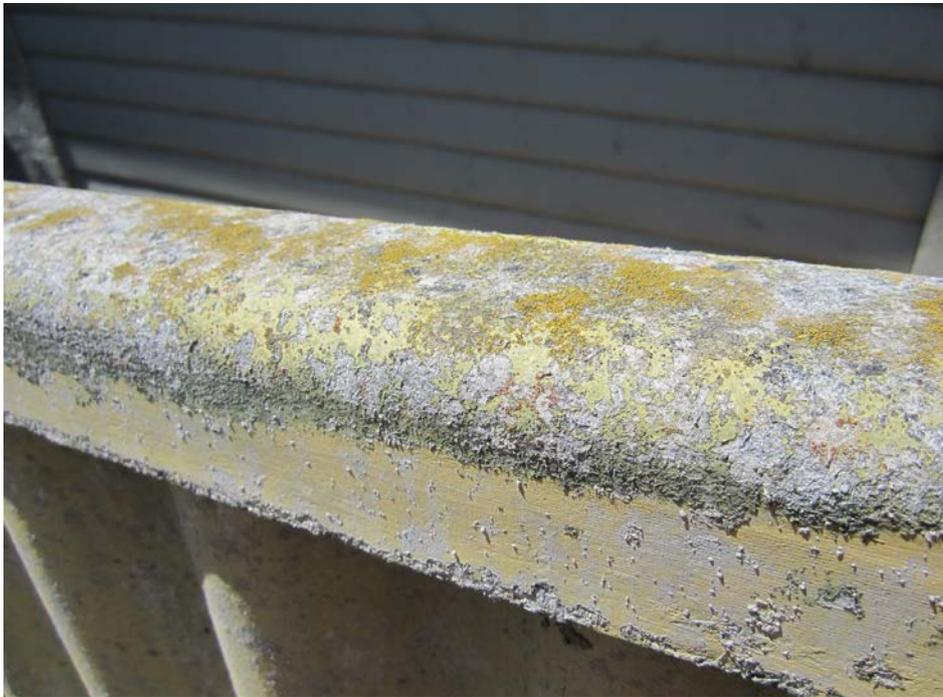
Photo 15. Mould (orange and green) on old painted (yellow) ACM capping
