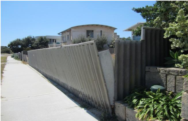
Photo 10. Collapsing ACM fence
