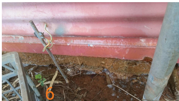
Outflowing water leak from within the Kitchen wall
